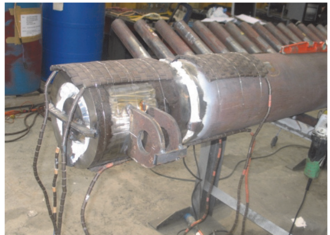
Fig 3 – Gr 91 header repair showing weld, purge and preheat set up
