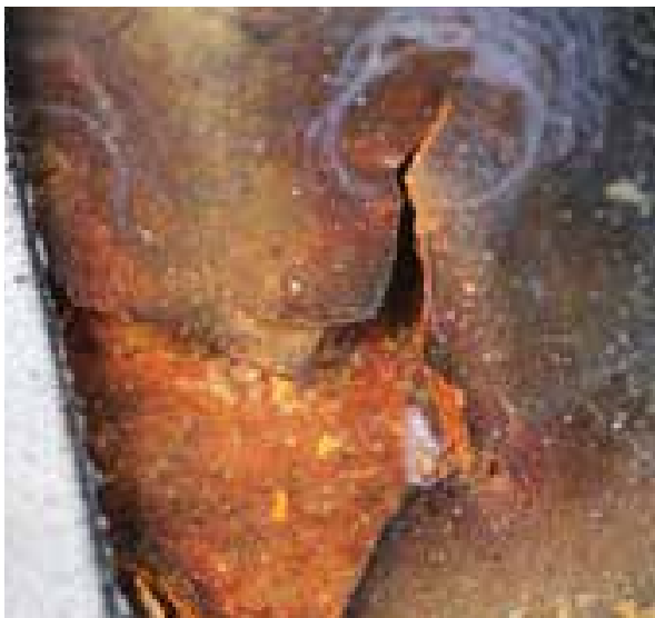
Fig. 3 Cracking due to residual stress
